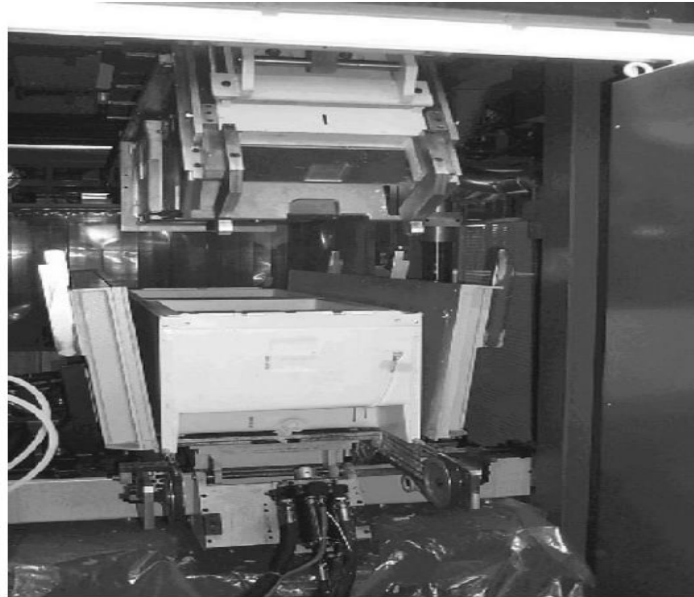
Figure 13 - Example of a foaming machine and mold for refrigerators
